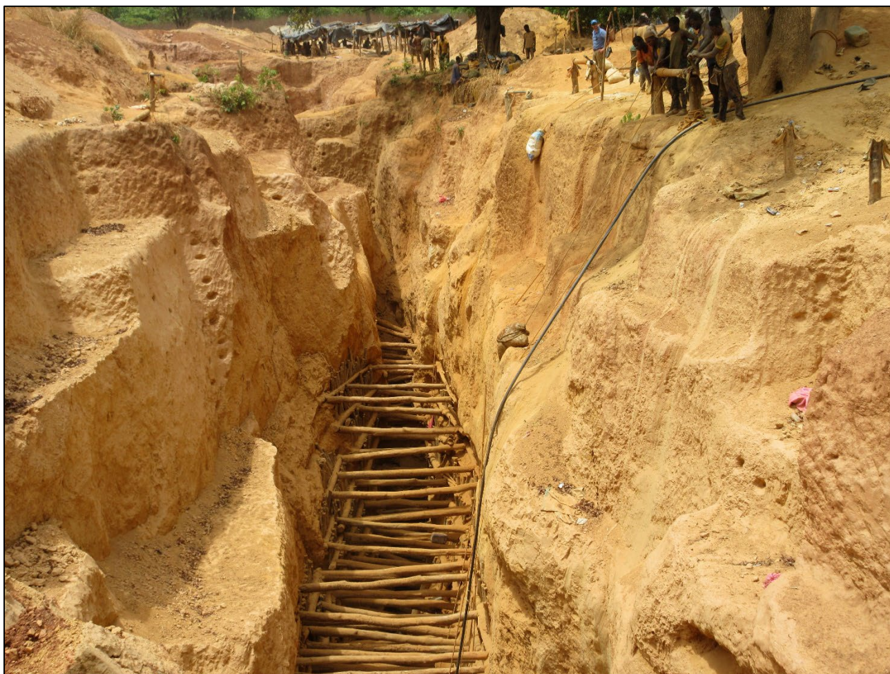
Figure 3: Tchaga North - Deep artisanal mining site on western contact of greenstone and granite – location is shown on Figure 1
